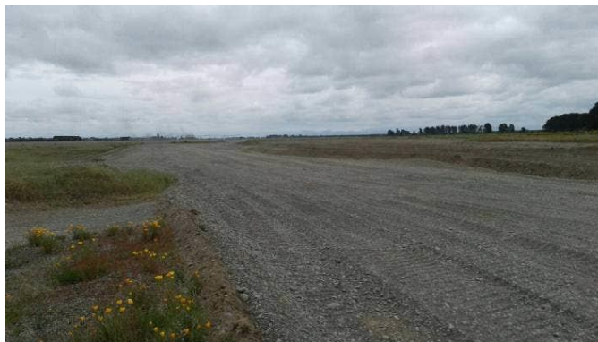
A development on the Selwyn Riverbed. A local dairy farmer was served an abatement notice
